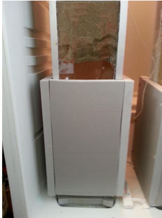
Fig.2 Thermally insulating by extruded polystyrene shields
